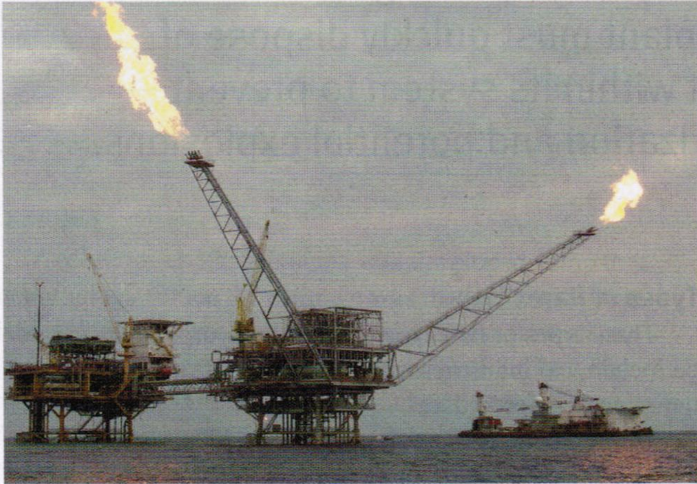
▲ Figure 3. Other multi-point flare systems are elevated.
